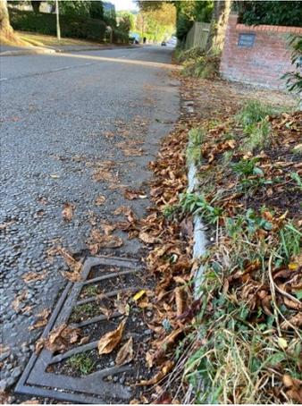
This is a familiar picture of a drain (or gully at HCC call it) as Autumn progresses: leaves and muck washed into it creates a solid block which stops further water draining away.
